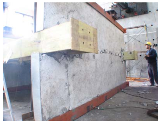
Figure 5. Crack at the top slab
